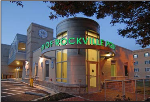
Rockville Police Department Headquarters City of Rockville, MD
