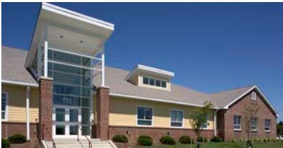
Queen Anne's County Office Building Centreville, MD
