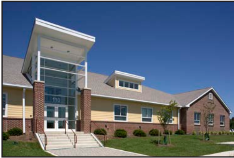
Queen Anne's County Office Building Centreville, MD
